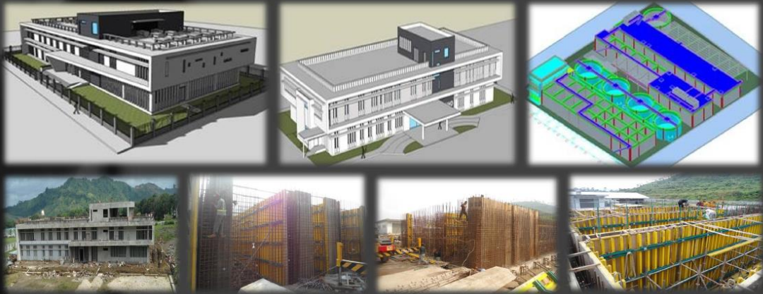
Construction for PT. Paiho Indonesia – Sukabumi 2012-2014
